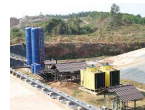
(Left) The palm oil mill operated by Krabi Oil-Palm Farmers Cooperatives Federation Ltd generates about 500 m 3 of palm oil mill effluent (POME) per day during its processing. This is piped online from the production to the KrabiWTE biogas plant built next door. The POME is received in the fat pit and cooling pond (centre) where fats, oil and grease (FOG) is removed and the temperature cooled before it is pumped into the modified Anaerobic Baffle Reactor (ABR). The raw biogas from the ABR is then passed through a cleaning unit (right) to remove impurities before it goes to the gas gen-set.
