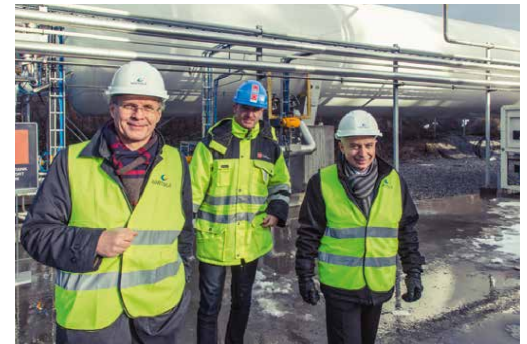
(Top) View of the Wärtsilä biogas liquefaction plant at EGE Biogass during the official opening. Key components are (1) the LBG control system, (2) the glycol pre-chiller, (3) the raw biogas pre-treatment unit, (4) the liquefaction unit and (5) the onsite LBG storage and export station. The bus used ran on biogas too.
