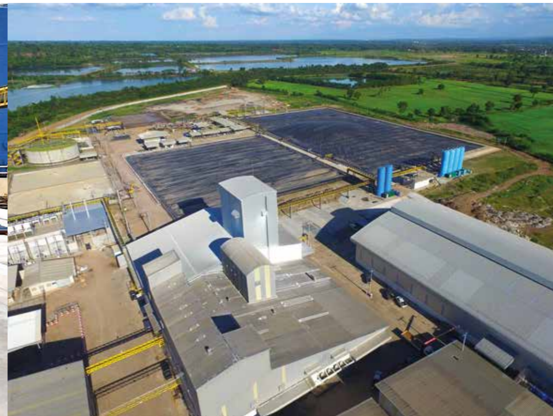
(Above left) An aerial view of the General Starch plant at Chonburi, Thailand. Light Blue Bioscrubbers are shown in the foreground before the gas is used in MTU CHP sets. Four large flares located the back of the site as well as the SCADA PLC control system, Laboratory and Control Building. (Above right) Dr Ulrike Leroff advising on granule formation at an Upflow Anaerobic Sludge Blanket Reactor at Chok Yuen Yong Plant in Nakorn Ratchasima (photos courtesy Biotrix).
