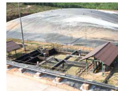
(Left) The palm oil mill operated by Krabi Oil-Palm Farmers Cooperatives Federation Ltd generates about 500 m 3 of palm oil mill effluent (POME) per day during its processing. This is piped online from the production to the KrabiWTE biogas plant built next door. The POME is received in the fat pit and cooling pond (centre) where fats, oil and grease (FOG) is removed and the temperature cooled before it is pumped into the modified Anaerobic Baffle Reactor (ABR). The raw biogas from the ABR is then passed through a cleaning unit (right) to remove impurities before it goes to the gas gen-set.
