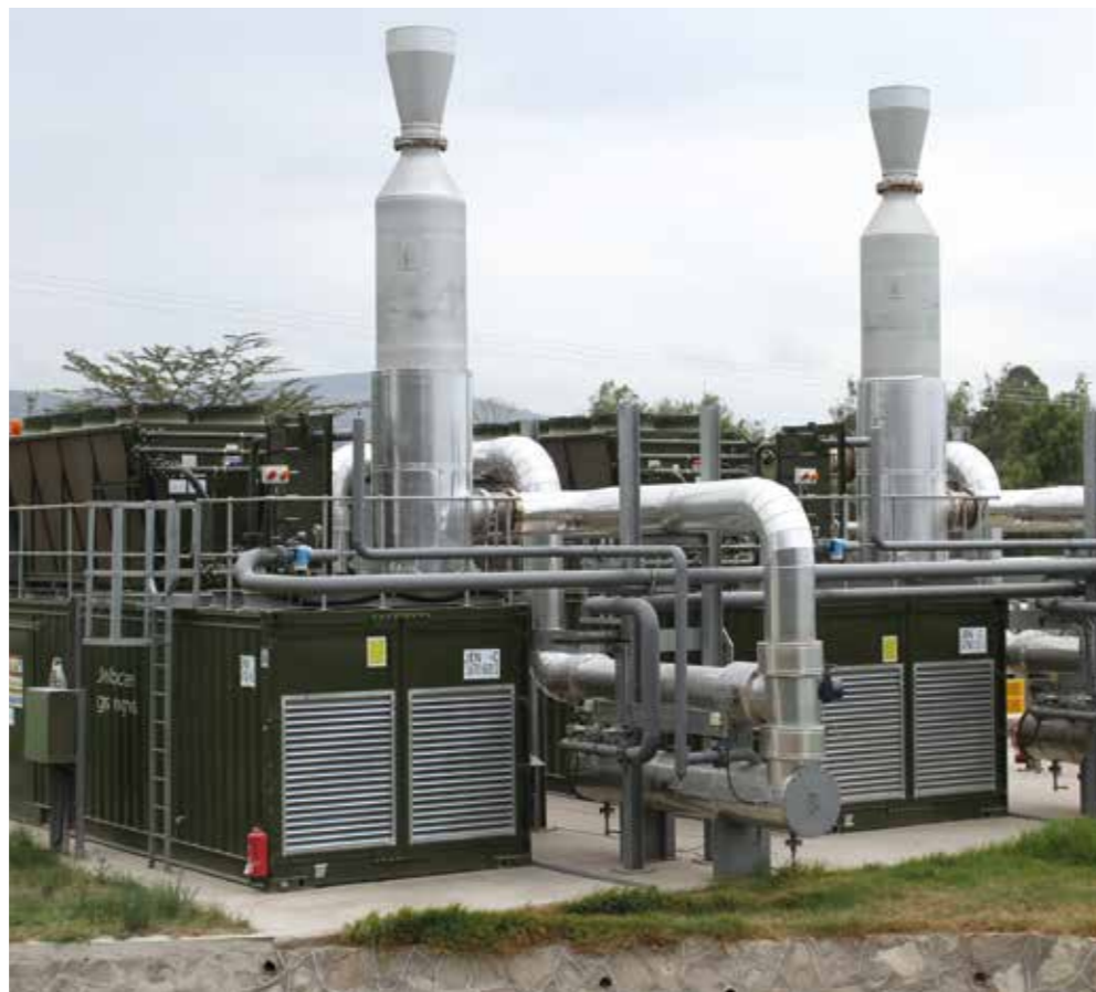
(Above) The biogas is used to fuel two self-contained GE Jenbacher 420 gensets. The engine and exhaust heat is recovered to support the biogas process and to heat nearby plant propagation houses. Nighttime temperatures can be quite cool at 2 km above sea level and roses love a steady 22 degrees.
