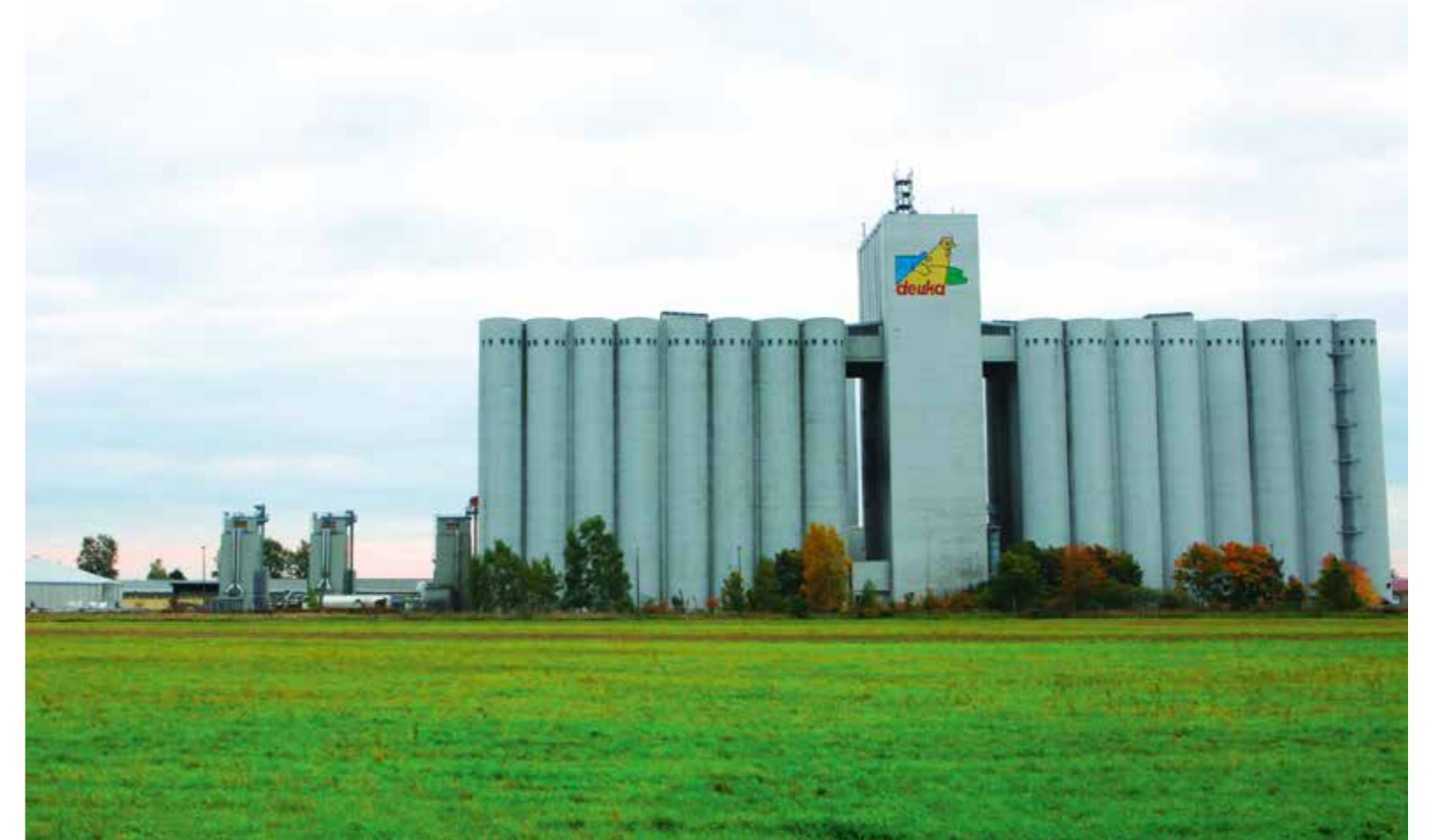
The biogas plant (left) is located next door to the Deutsche Tiernahrung Cremer animal feed facility in Herzberg, Germany. Cremer provided the site and leased it to EnviTec who financed and built the biogas plant. The plant supplies heat in the form of hot water and saturated water vapour to Cremer.
