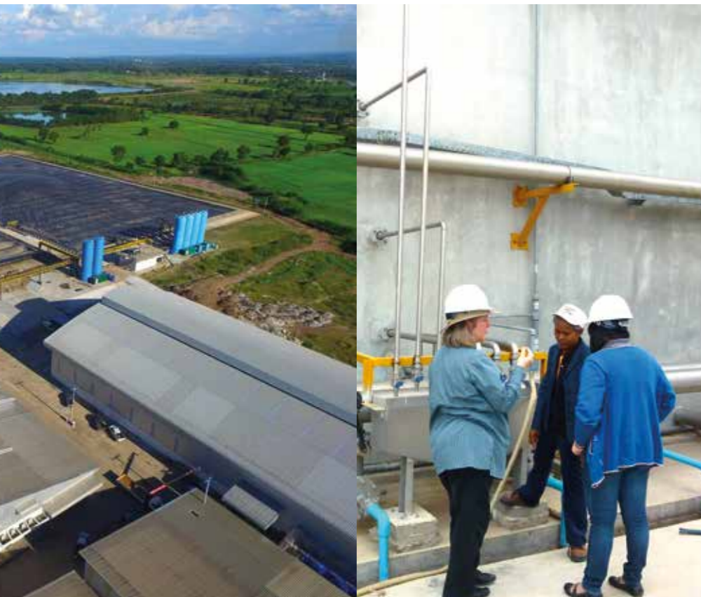
(Above left) An aerial view of the General Starch plant at Chonburi, Thailand. Light Blue Bioscrubbers are shown in the foreground before the gas is used in MTU CHP sets. Four large flares located the back of the site as well as the SCADA PLC control system, Laboratory and Control Building. (Above right) Dr Ulrike Leroff advising on granule formation at an Upflow Anaerobic Sludge Blanket Reactor at Chok Yuen Yong Plant in Nakorn Ratchasima (photos courtesy Biotrix).
