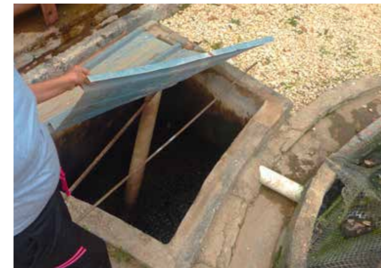
Taking a closer glance into the fermenter. After the digesting process the raw biogas is pumped from the fermenter to storage and the cooperative kitchen.
