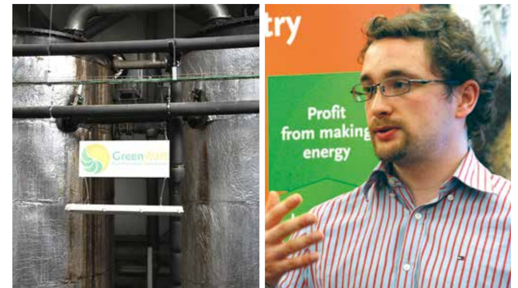
The HYFAD reactor consists of two well insulated 25m 3 vessels keeping a temperature of 38°C and neutral pH. It produces 75 percent of the biogas.
